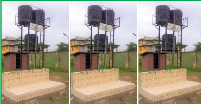
SEMI-INDUSTRIAL BOREHOLE AT INIKOROGHA COMMUNITY
