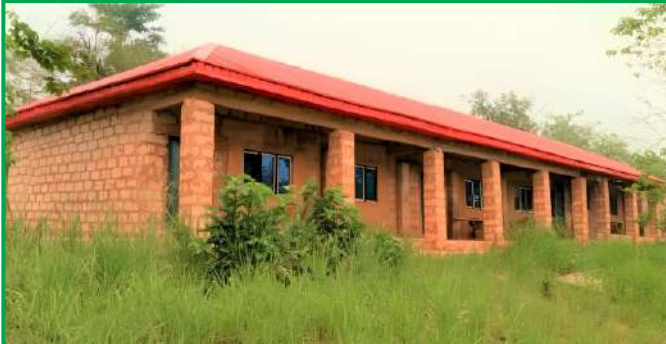
FIRST PHASE OF THE CONSTRUCTION OF A BLOCK OF CLASSROOMS AT ORHUA COMMUNITY
