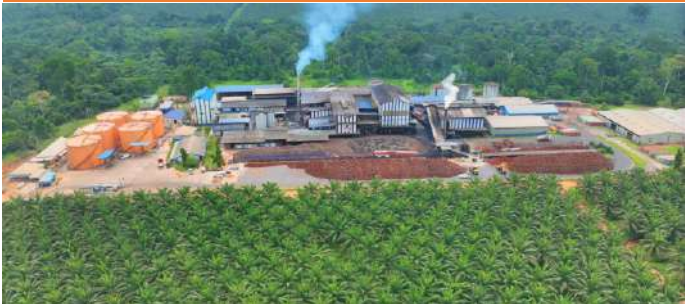
AERIAL VIEW OF THE MAIN ESTATE OIL MILL AND PLANTATION
