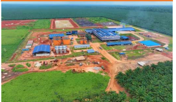
AERIAL VIEW OF THE COMPLETE 60T/HR OIL MILL AND PLANTATION OFFICE AT EXTENSION 2 IN 2023
