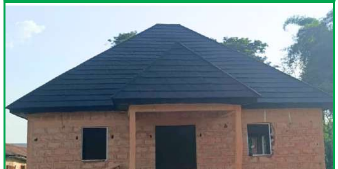
FIRST PHASE OF THE CONSTRUCTION OF MATERNITY HOME AT EKPAN COMMUNITY
