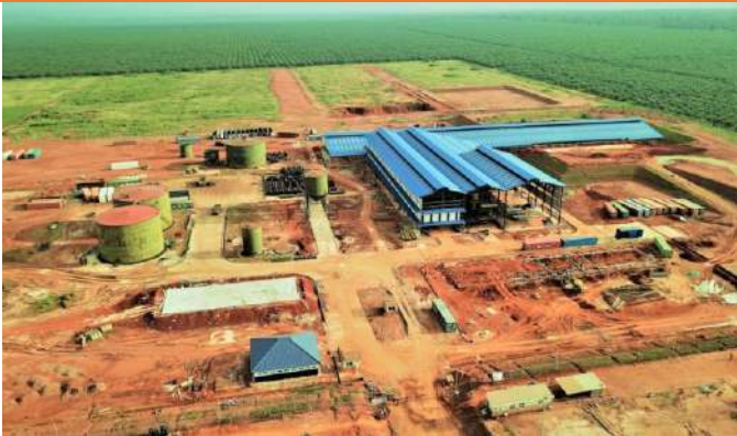
CONSTRUCTION OF OUR FIRST 30T/HR OIL MILL AT EXTENSION 2 IN 2020
