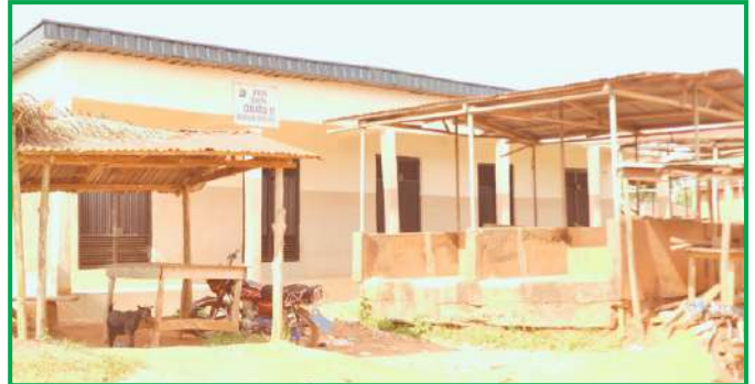
A BLOCK OF MARKET STALLS BUILT AND DONATED TO TRADERS IN UMOKPE COMMUNITY
